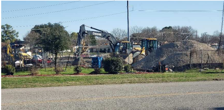
Corner Stone Plaza Construction
