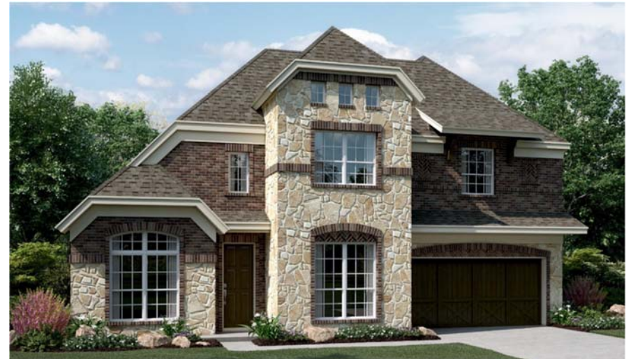
Oakdale Homes Celina, TX
