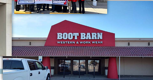
Boot Barn exterior improvements
