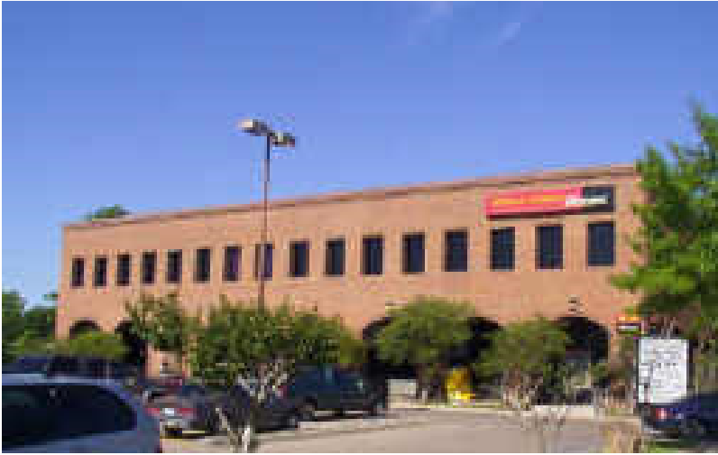
120 W Main St. – General Office
