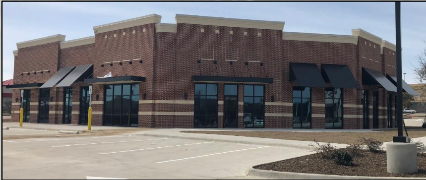
New retail and office facility on Belt Line Road near US Hwy. 80
