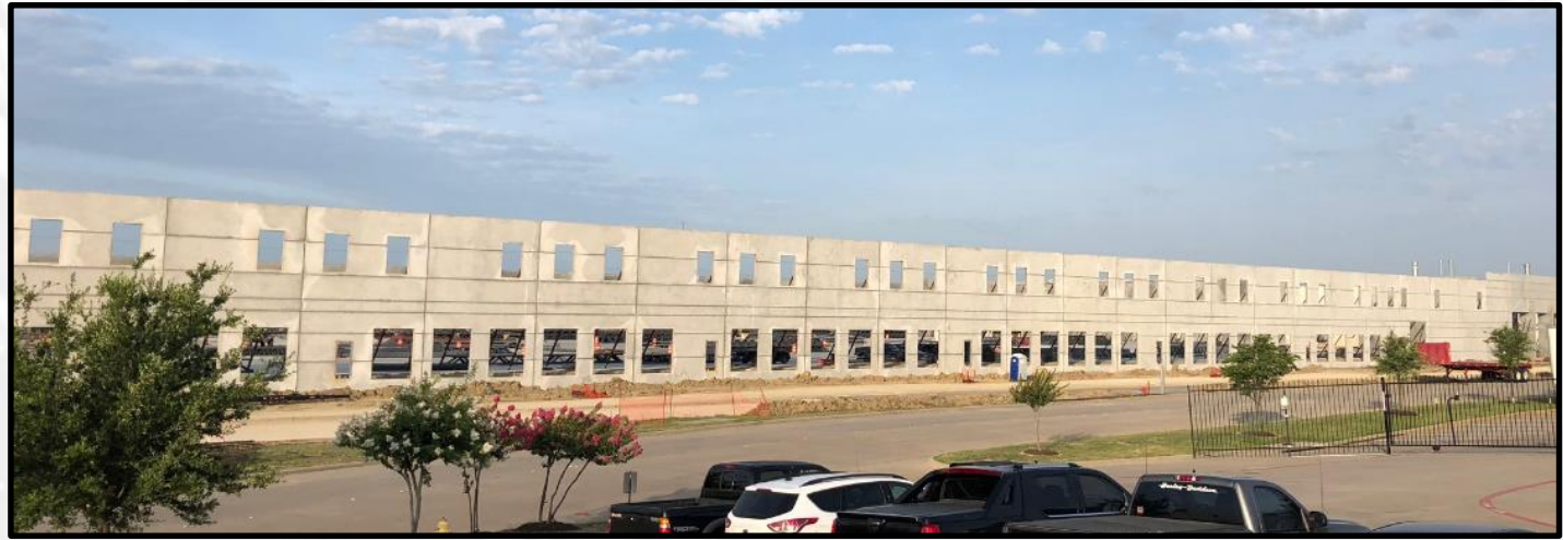
IDI Building D during construction in Skyline Trade Center
