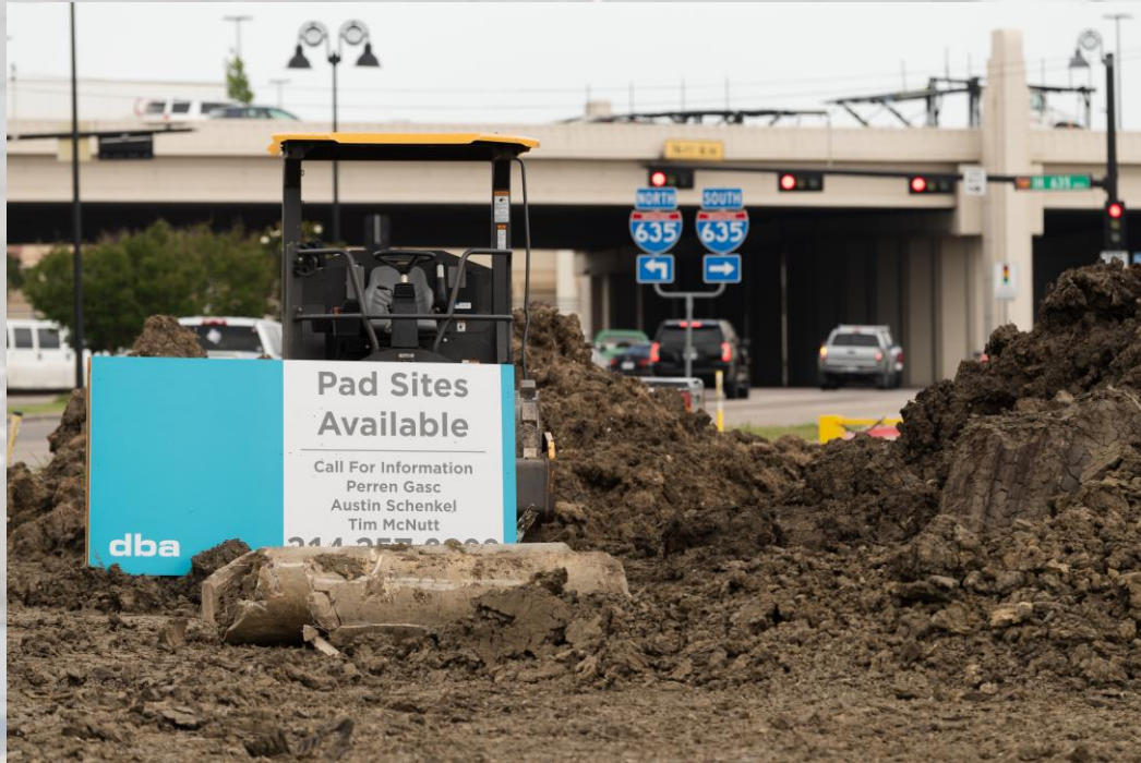
Project Stallion begins site work for five new pad sites
